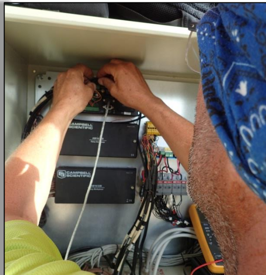
Automatic recording of TDR probes and sap flow sensors.
