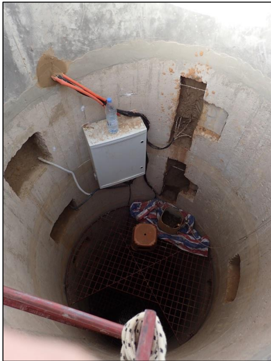
Automatic scanners, suction caps and TDR probes set up down to the water table (-6 m).
