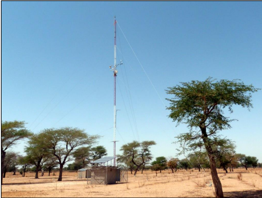
Eddy-covariance antenna (30m) + shelter (4.5 m 2 ) + fence + solar panels (4.5 m 2 ) + Campbell weather station +GNSS.
